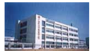
Hitachi Air Conditioning & Refrigerating, Китай
